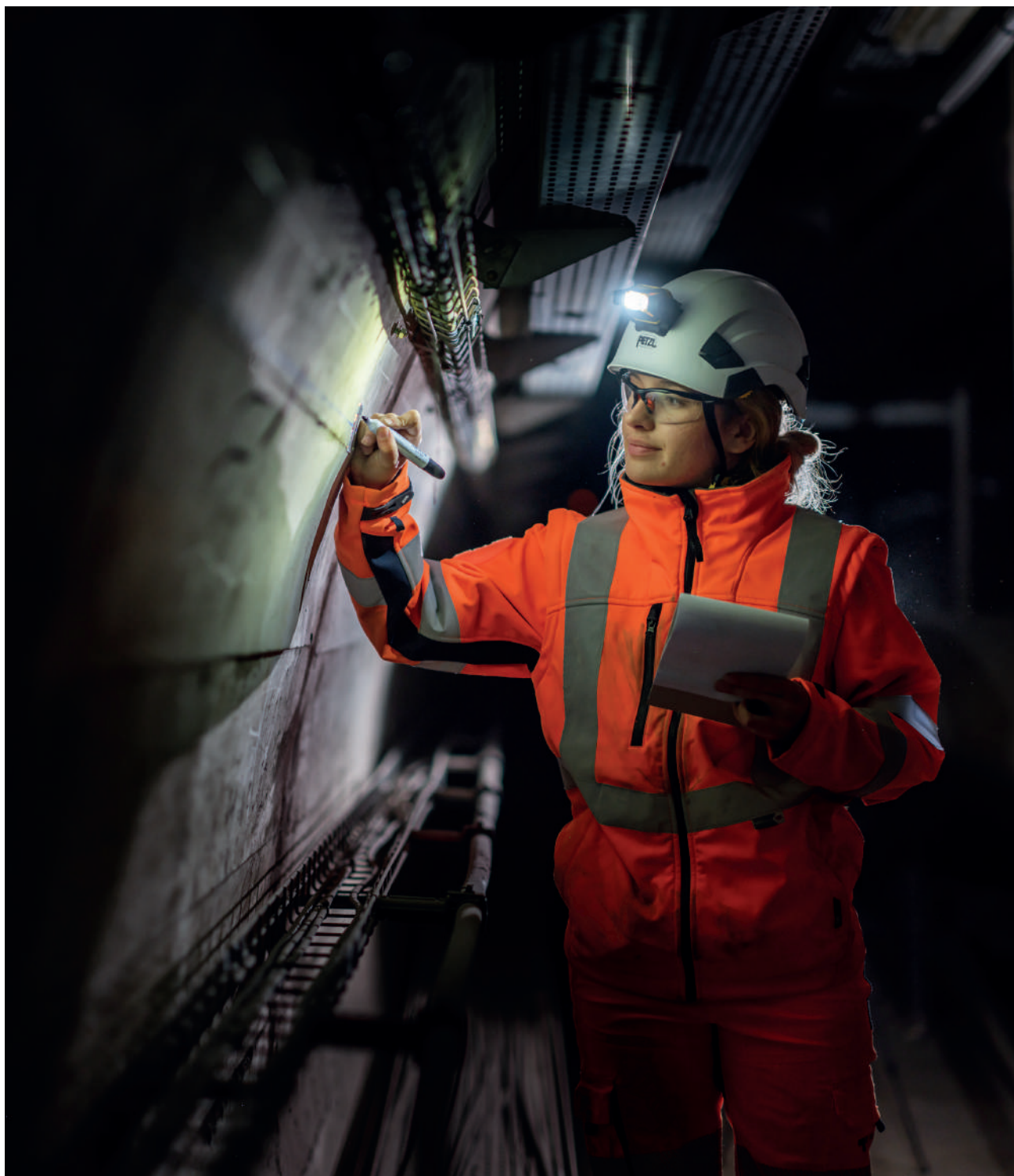
Underground structural monitoring, Paris, France © 2024 Petzl Distribution - Rémi Flament - Novatias
